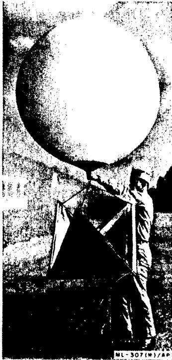
Figure 50. Pilot Balloon Target ML-307/AP or ML-307A/AP ready for flight.
