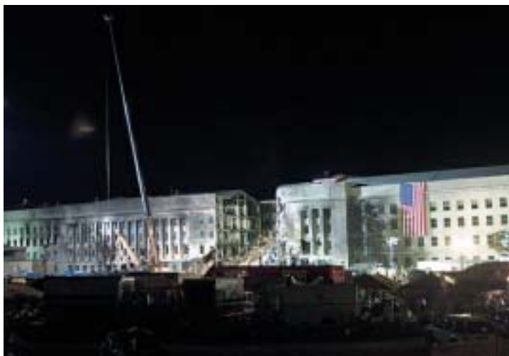
The portion of the Pentagon hit by a hijacked airplane on September 11, 2001, was illuminated as round-the-clock recovery efforts continued.
