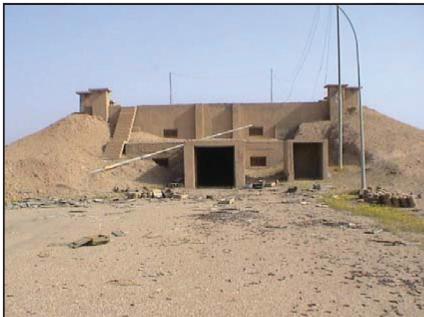
Figure 29. Small bunker with lightning protection.
