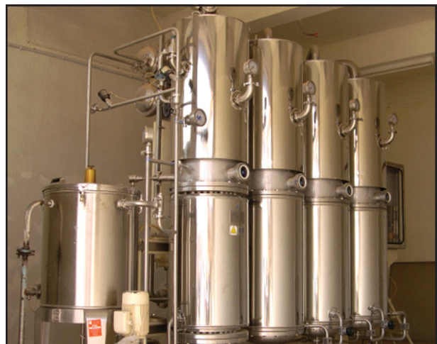
Figure 8. High grade water production plant.
