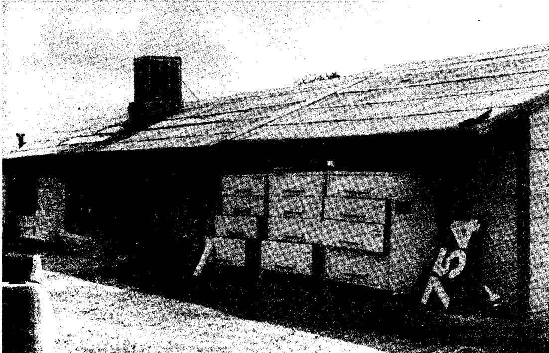
Figure 20. Building 754 as a Golf Course storage facility in 1996 prior to demolition, north and east elevations.
