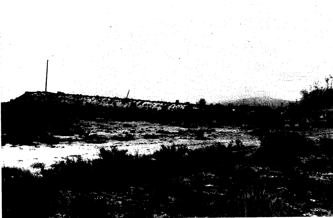
Figure 74. JB-2 Ramp in 1995, west profile (HAFB Environmental Flight, Cultural Resources Photo Archives).
