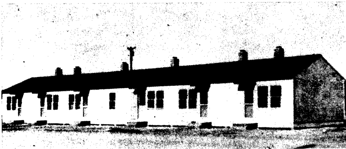
Figure 13. Typical theater-of-operations (TO)-type temporary structure at AAAF, “Alta Vista Civilian Housing, Girl’s Dorm” (Alamogordo Army Air Base [1942]).
