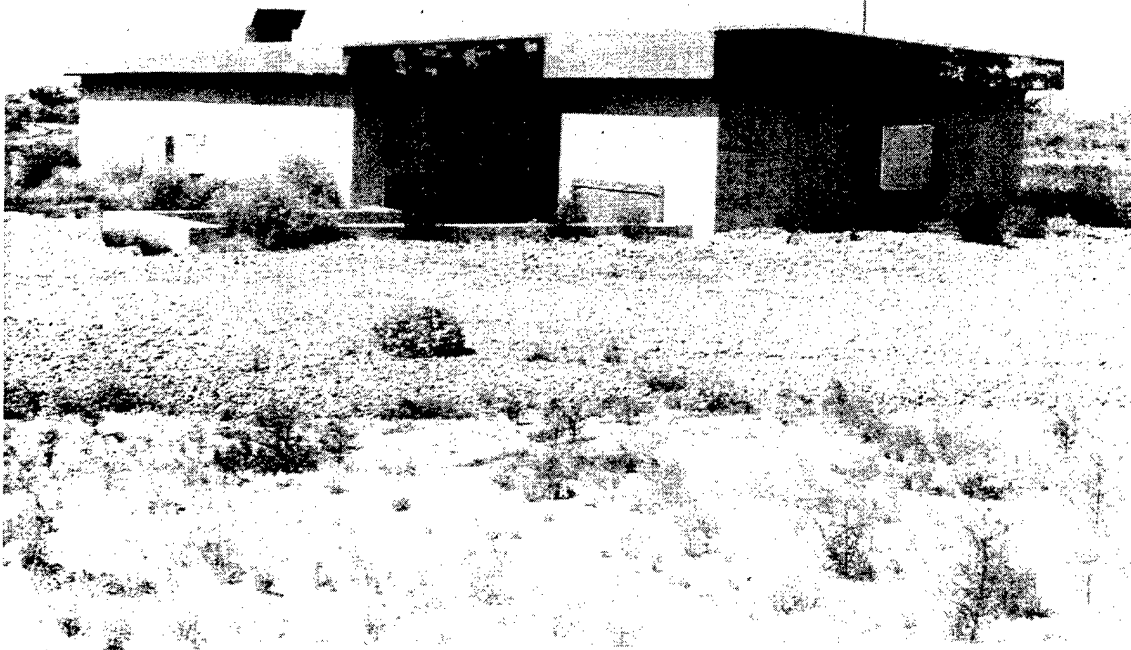
Figure 98. Building 1113 as a Dynalectron Corporation storage facility in 1996, northeast and southeast elevations.
