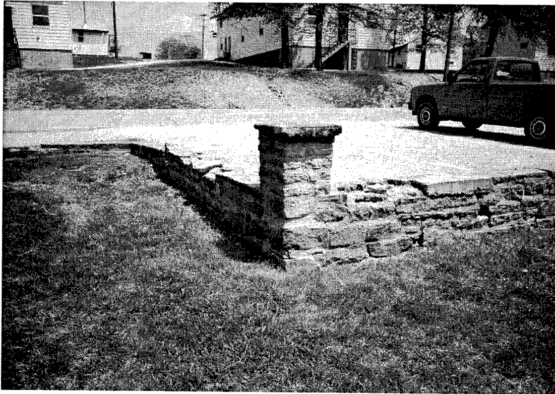
Figure A-4 Corner of Wall in Front of Building 2101 (courtesy, DPW Fort Leonard Wood).
