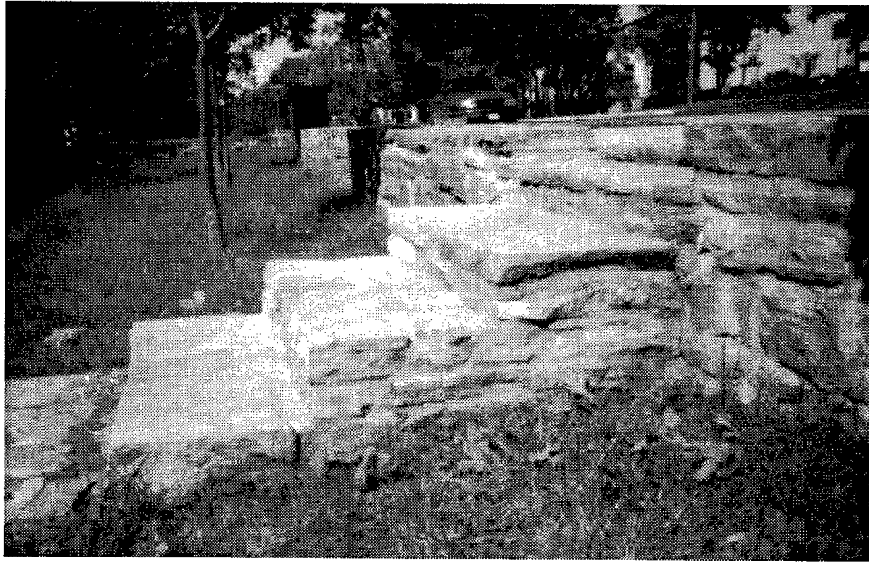
Figure A-3 POW Stonework Steps, Building 2101 (SCIAA).
