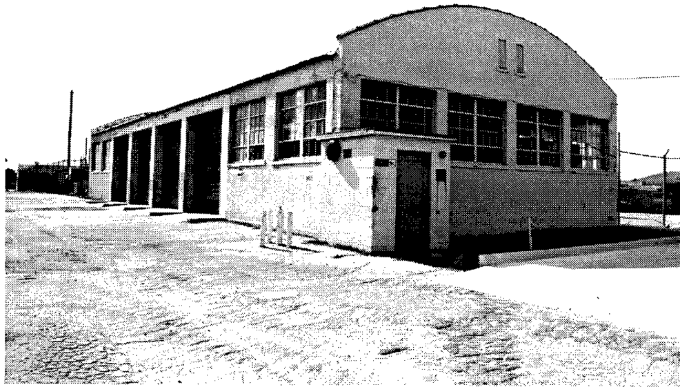
Figure 29. 1994 photo of Building Number 2952; continues to serve as a motor repair shop (vehicle maintenance).
