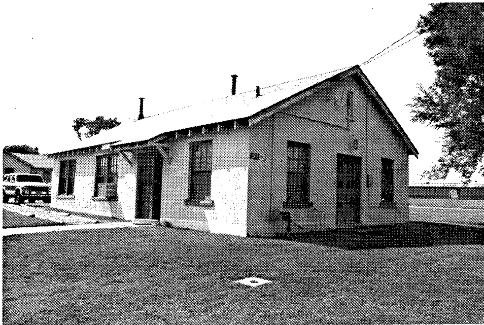
Figure 20. 1994 photo of Building Number 2919; originally constructed as a regimental headquarters building.
