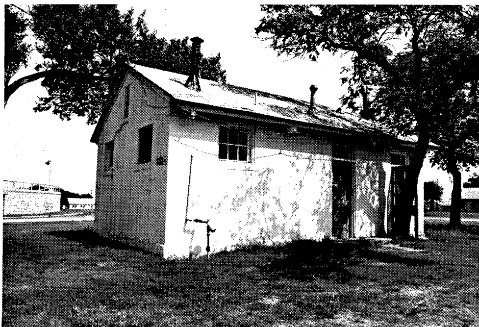
Figure 36. 1994 photo of Building Number 2925; continues to serve as a latrine.
