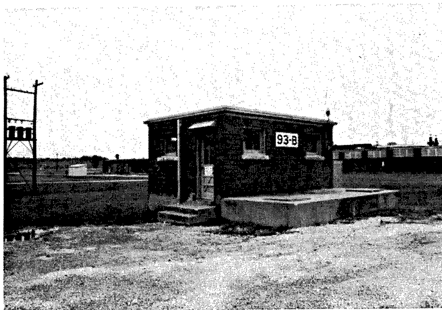
Figure 196. Building 93B: Industrial Waste Pump House.
