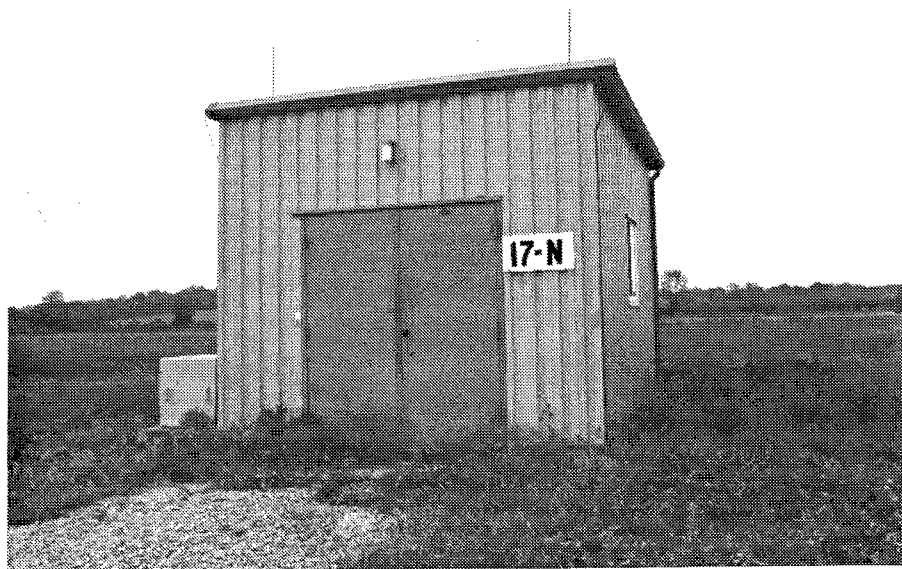
Figure 259. Building 17N: Well Pump Station.
