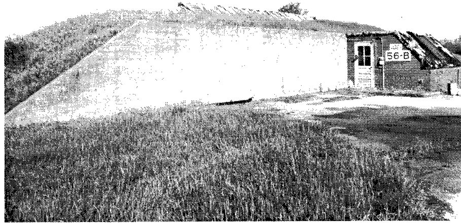
Figure 186. Building 56B: Firing Range Observation Building.
