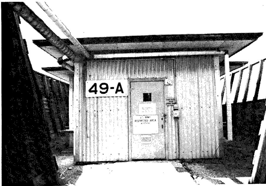
Figure 146. Building 49A: Primer Drying and Storage Building.
