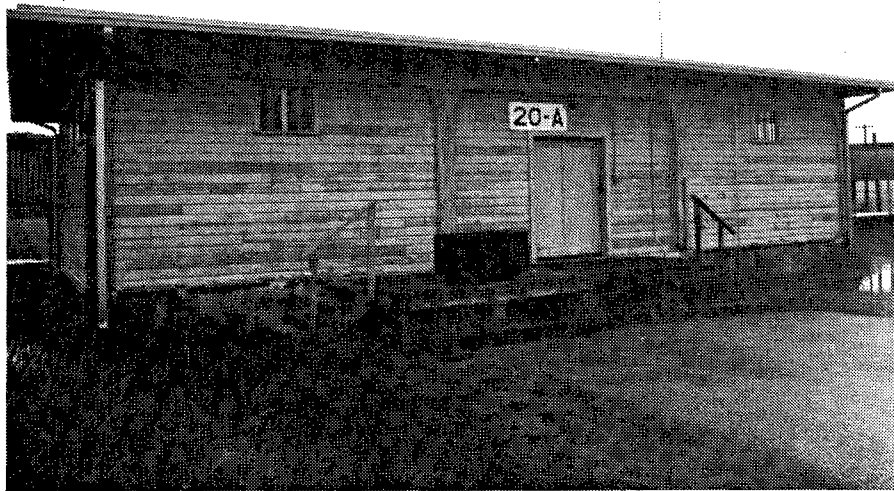
Figure 209. Building 20A: Empty Powder Case Storage Magazine.
