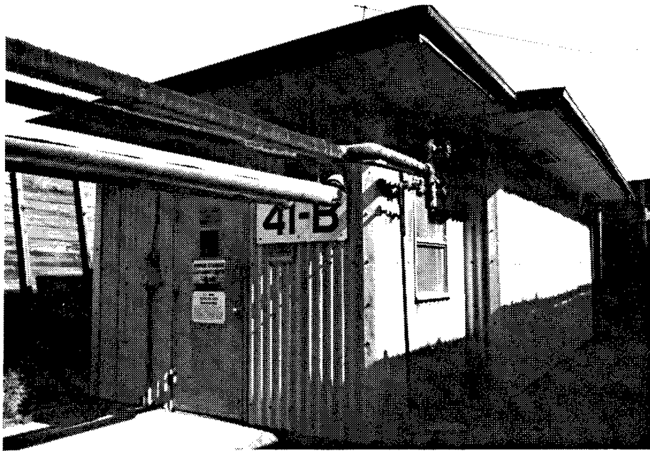
Figure 142. Building 41B: View of a Primer Drying and Storage Building.
