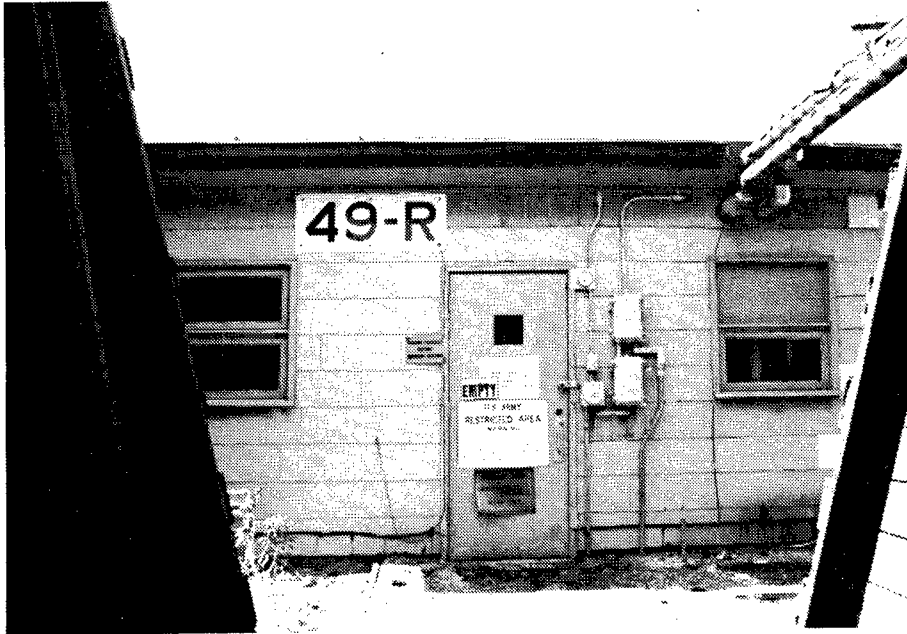
Figure 145. Building 49R: Primer Drying and Storage Building.
