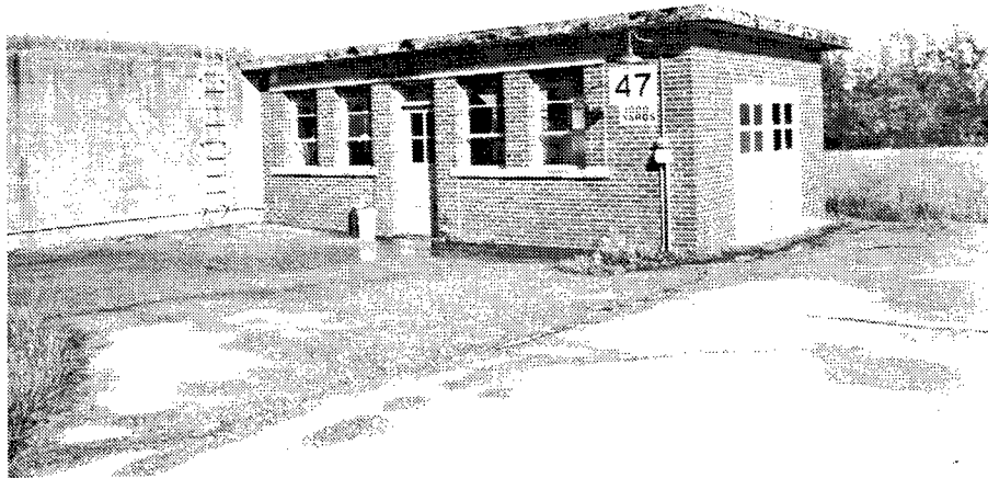
Figure 180. Building 47: Firing Range Target Storage Building.
