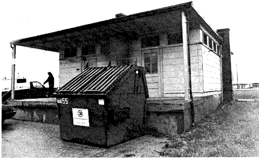
Figure 225. Building 32C: Primer Mix Area Change House.
