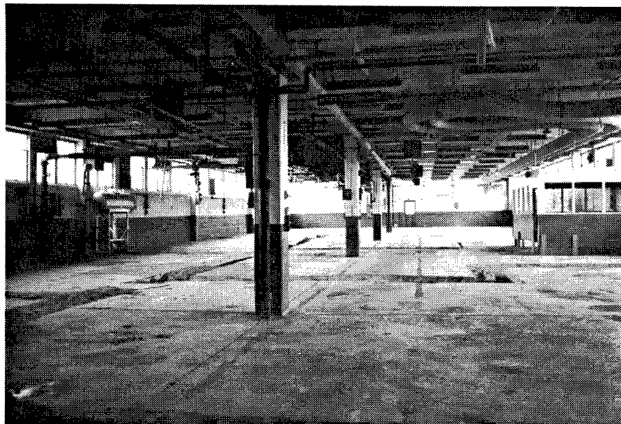
Figure 109. Building 12A: Interior of empty Fuze and Metal Parts Manufacturing Building.
