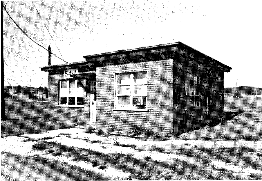
Figure 228. Building 54A: Change House and Attendant's Station.
