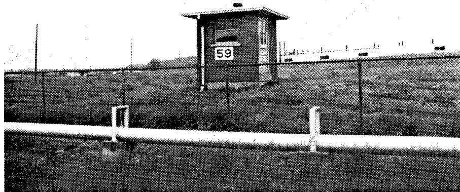
Figure 265. Building 59: Condensate Pump House for the Heating Plant.
