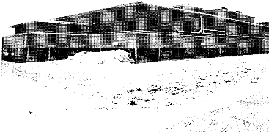
Figure 10. Building 2: 7.62 mm Ammunition Manufacturing Facility, Explosive Wing No. 1.
