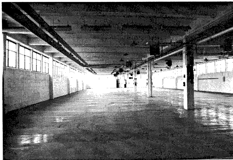
Figure 202. Building 7: Interior of empty General Storehouse.
