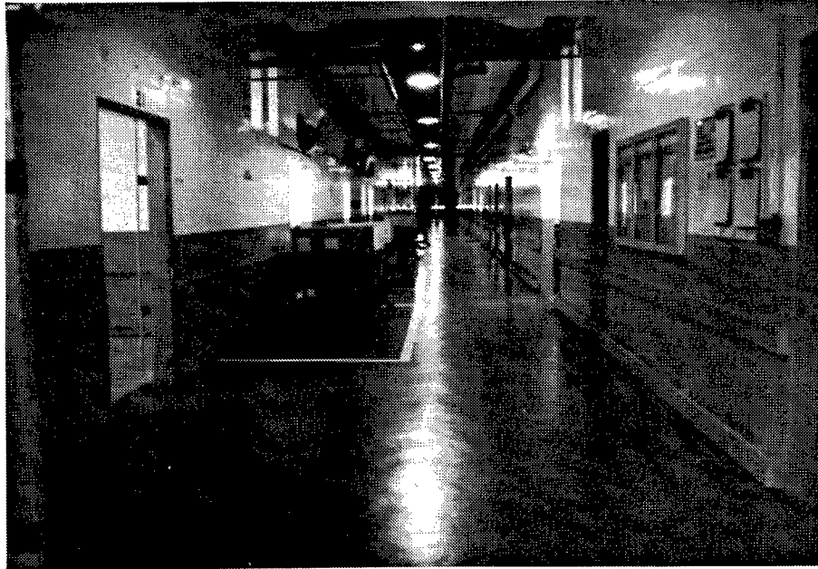
Figure 154. Building 65: Corridor dividing Bays.
