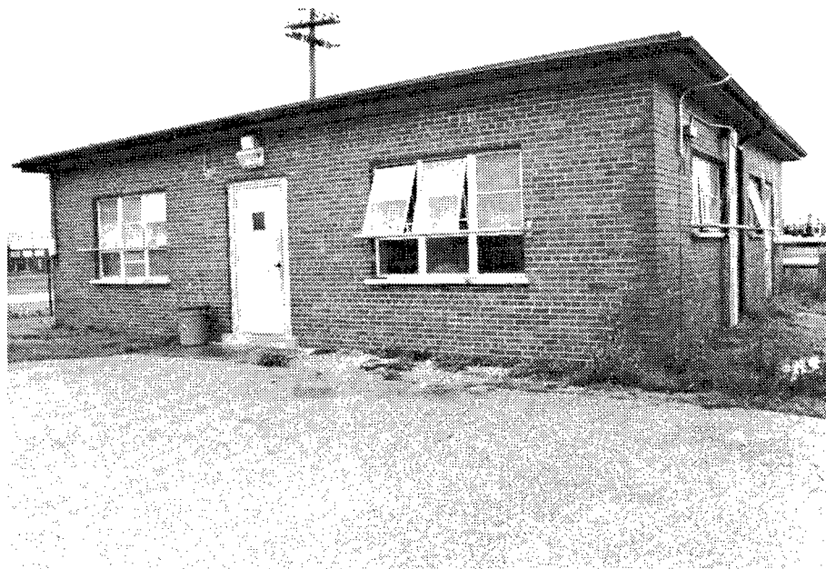
Figure 226. Building 53: High Explosive Pellet Area Locker and Change House.
