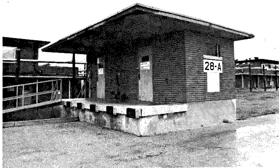
Figure 113. Building 28A: Tracer Chemical Distribution Building.
