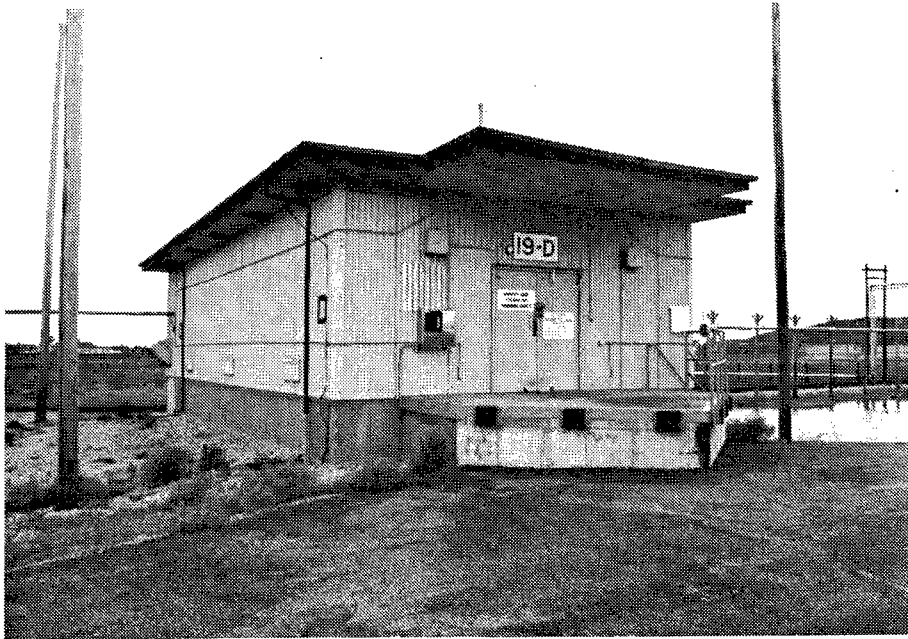
Figure 203. Building 19D: High Explosive Magazine for Powder Storage.
