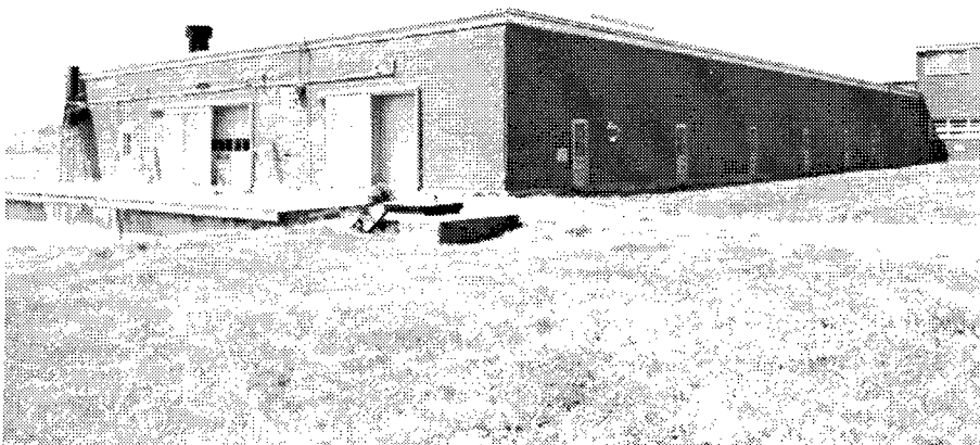
Figure 86. Building 3A: 20 mm Ammunition Manufacturing Facility, Explosive Wing No. 3.
