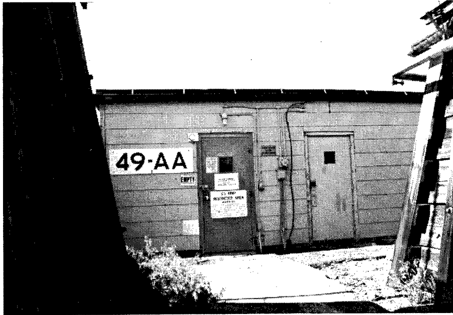
Figure 147. Building 49AA: Another view of a Primer Drying and Storage Building.
