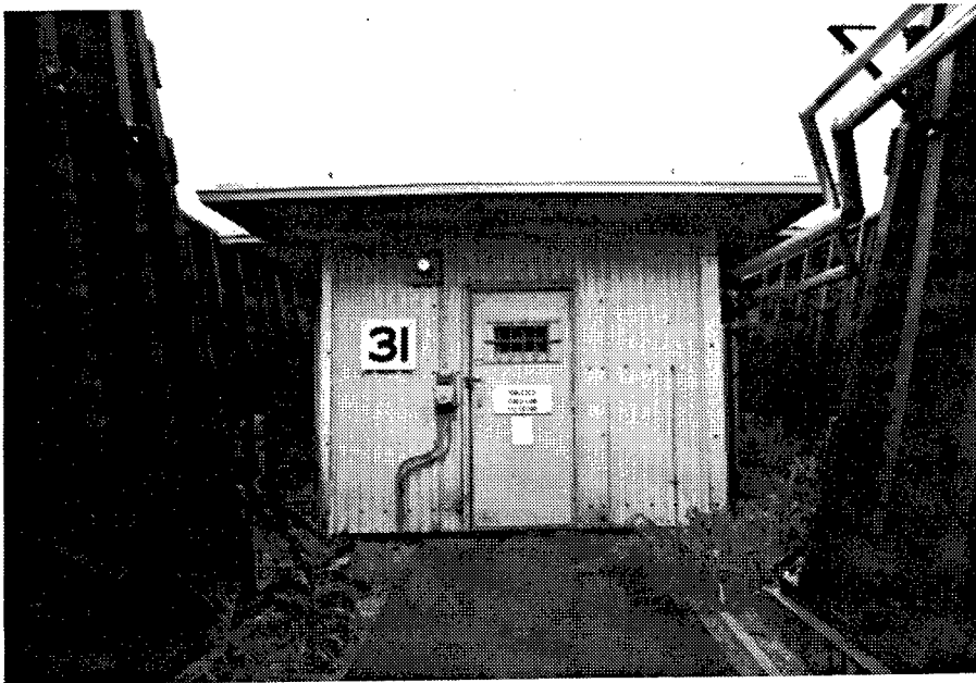
Figure 216. Building 31: Front view of High Explosive Pellet Storage Magazine.
