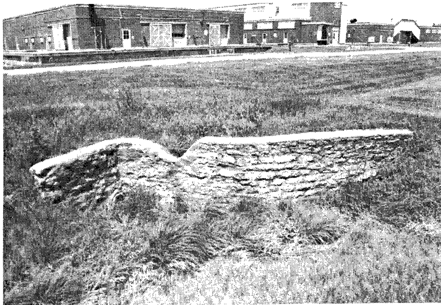
Figure 271. Culvert constructed in 1941.
