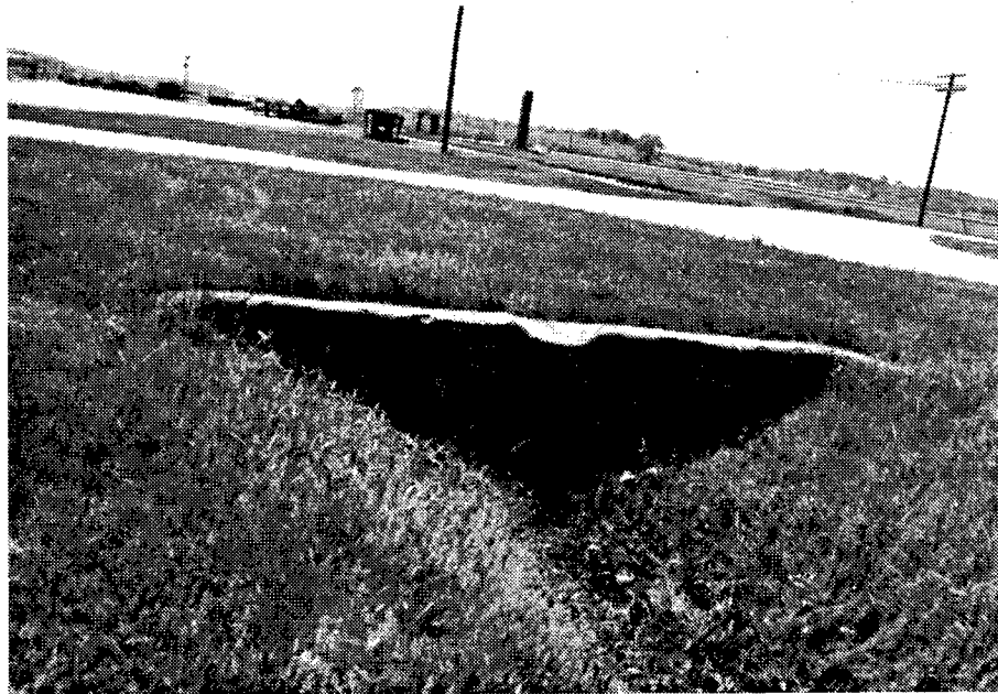
Figure 272. Another culvert constructed in 1941.
