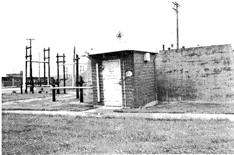
Figure 220. Building 37B: General Purpose Ammunition Storage Magazine.
