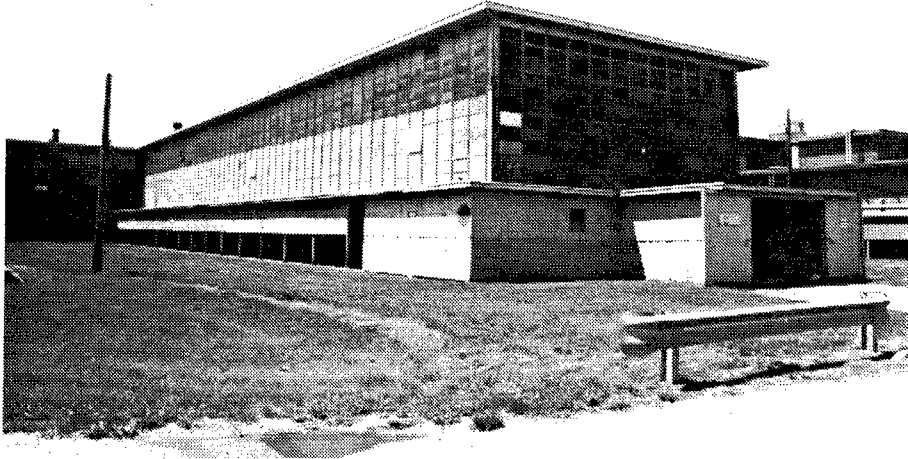
Figure 13. Building 2: 7.62 mm Ammunition Manufacturing Facility, Explosive Wing No. 3.
