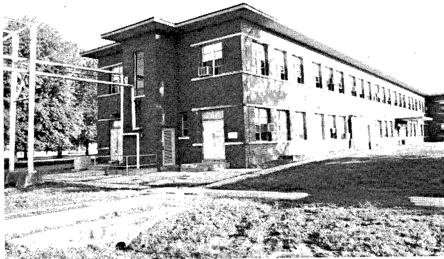
Figure 2. Building 5: Rear Wing of Administration Headquarters and Hospital.
