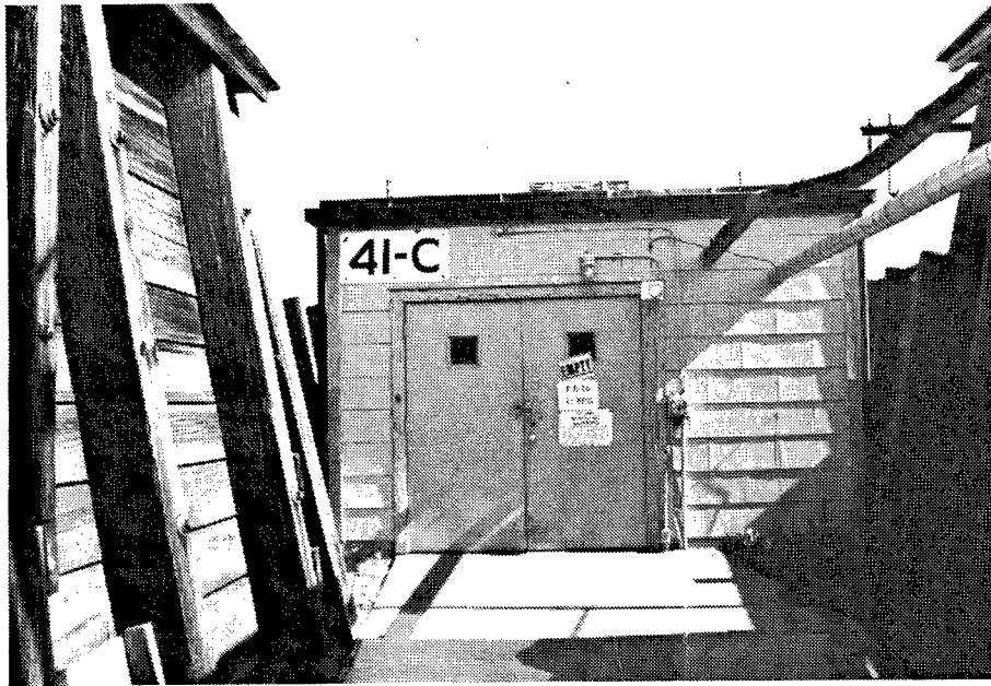
Figure 143. Building 41C: Primer Drying and Storage Building.
