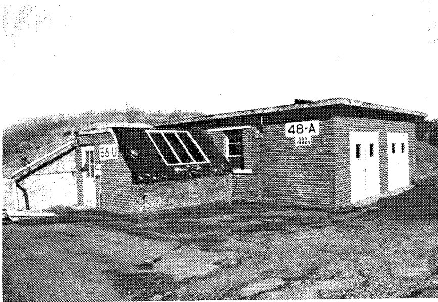
Figure 182. Buildings 48A and 56U: Firing Range Target Storage and Observation Buildings, respectively.
