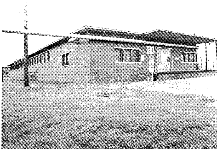
Figure 108. Building 12A: Fuze and Metal Parts Manufacturing Building.
