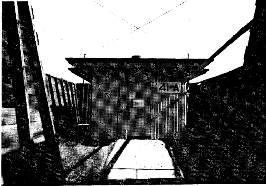
Figure 141. Building 41A: Primer Drying and Storage Building.
