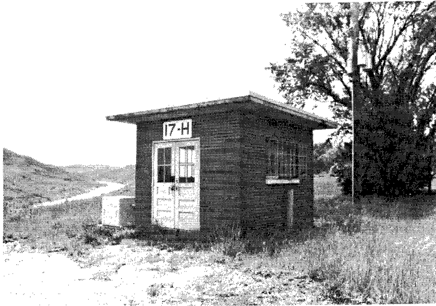
Figure 255. Building 17H: Water Booster Pump House.
