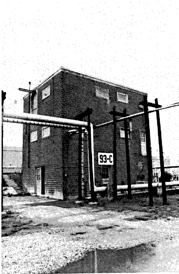
Figure 199. Building 93C: Industrial Waste Control Building.
