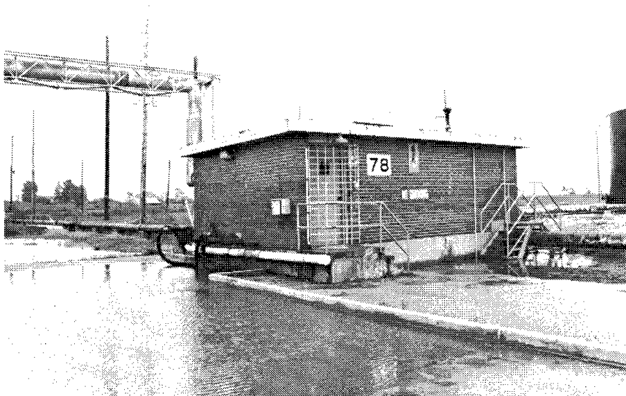
Figure 267. Building 78: Oil Unloading Pump House for the Heating Plant.
