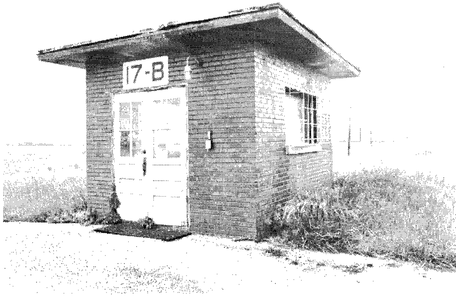
Figure 253. Building 17B: Well Pump Station.
