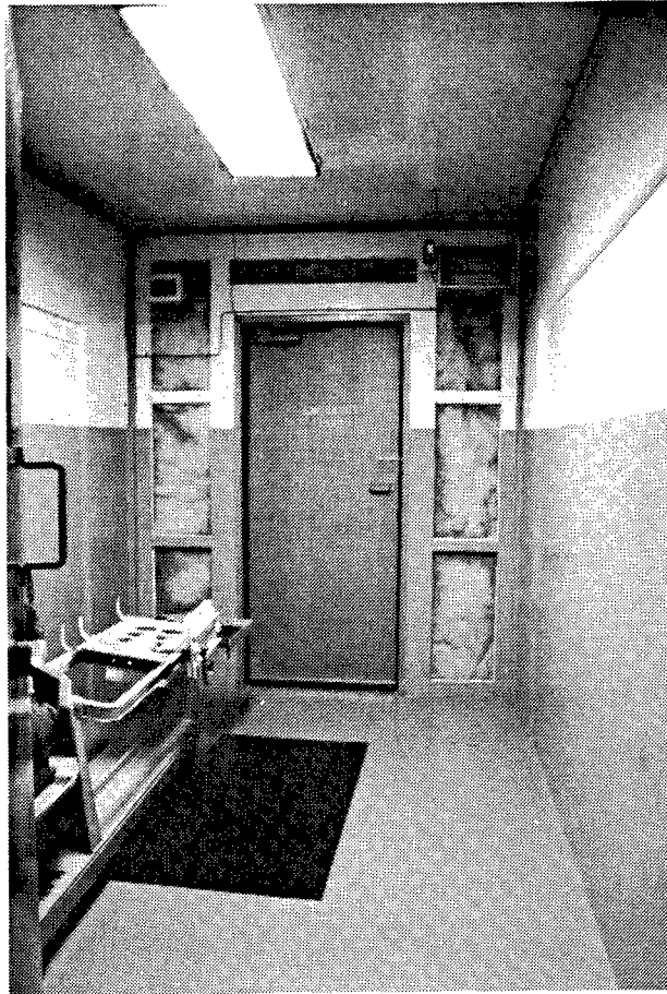
Figure 136. Building 38B: Blending Room.
