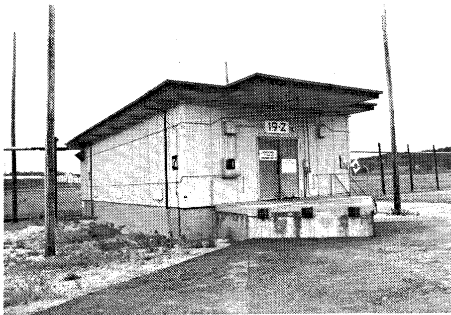
Figure 208. Building 19Z: High Explosive Magazine for Powder Storage.
