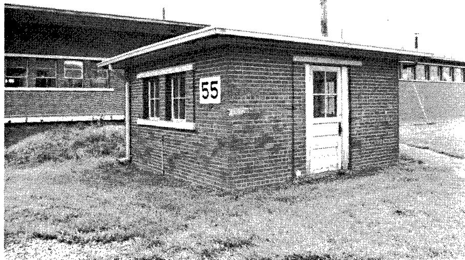
Figure 261. Building 55: Oil Unloading Pump House.
