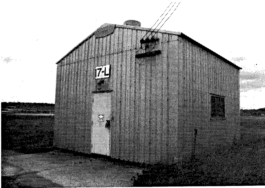
Figure 258. Building 17L: Booster Pump Station.
