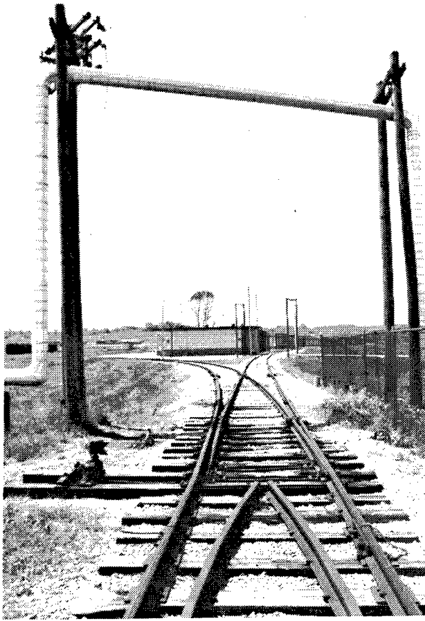
Figure 278. Railroad Tracks and Overhead Steam pipes.
