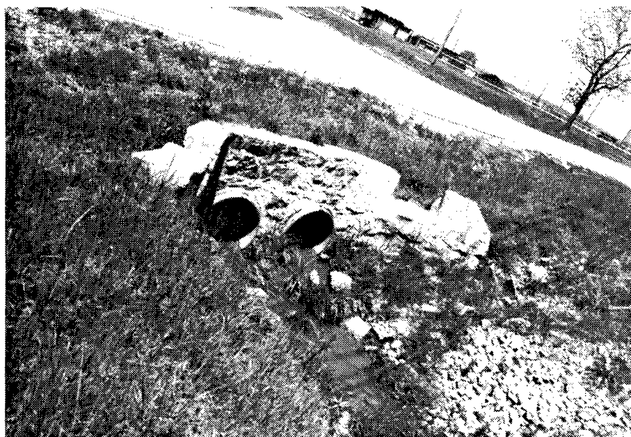
Figure 273. Culvert constructed in 1941.
