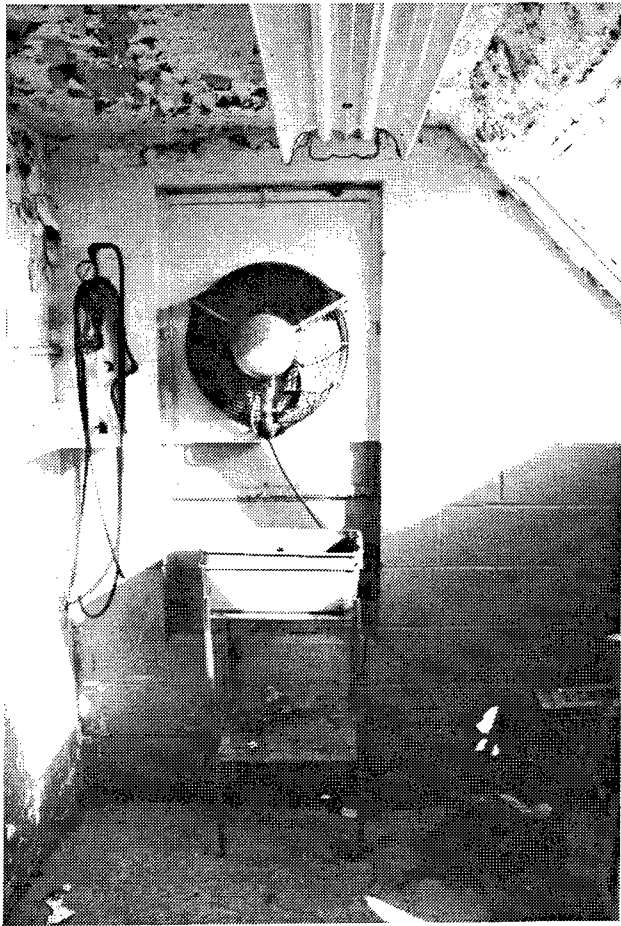
Figure 188. Building 56E: Interior of Firing Range Observation Building.
