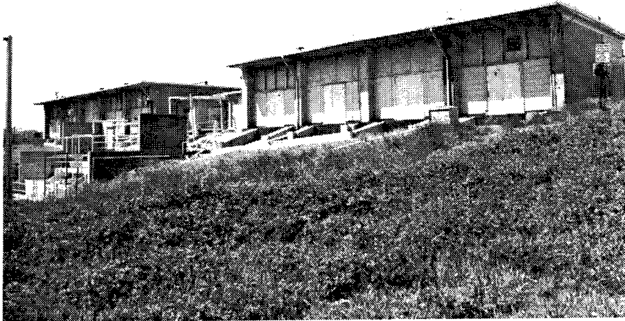
Figure 191. Building 81: Disposal Tanks Building.
