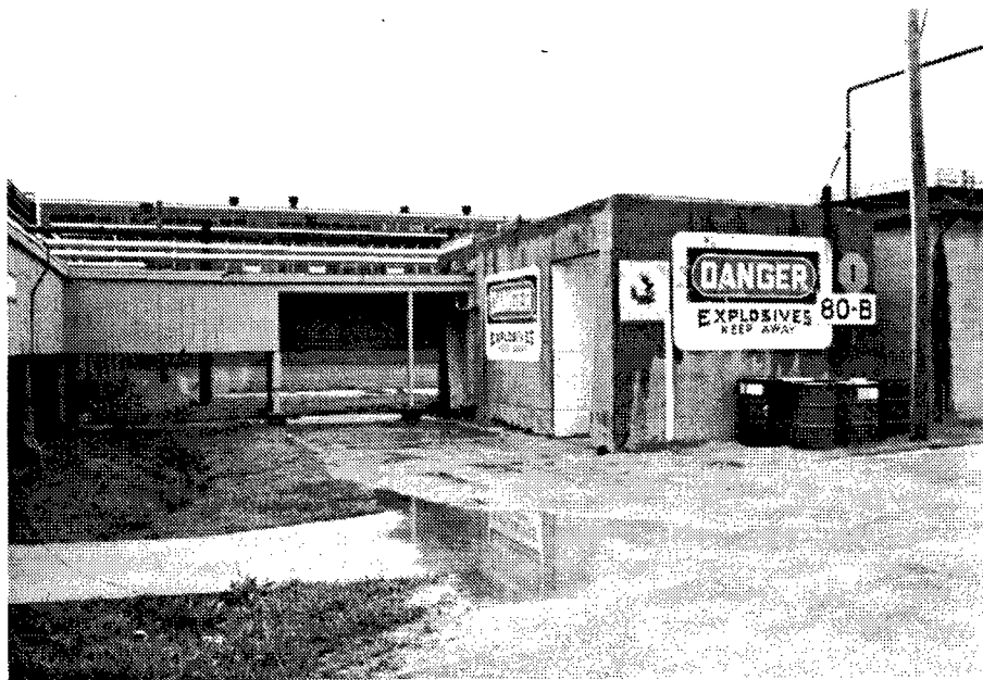
Figure 224. Building 80B: Pyrotechnic Storage Magazine.
