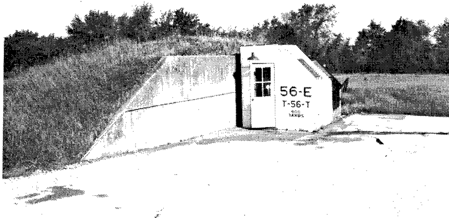
Figure 187. Building 56E: Firing Range Observation Building.
