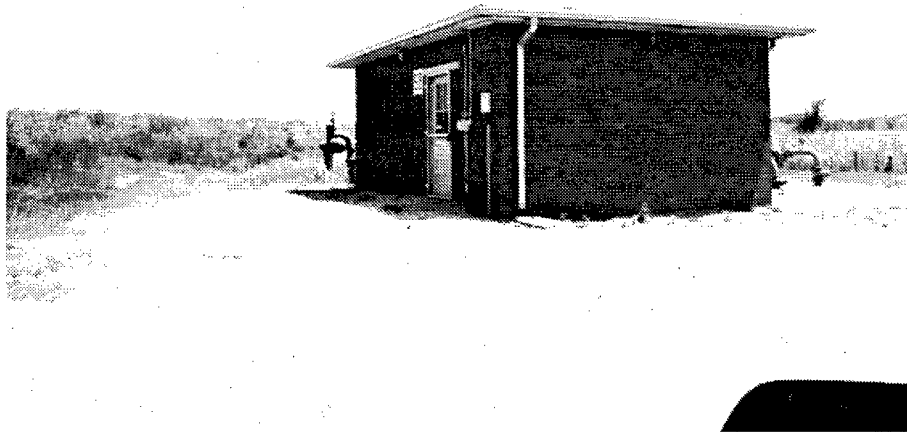
Figure 264. Building 58: Main Natural Gas Distribution and Master Meter House.
