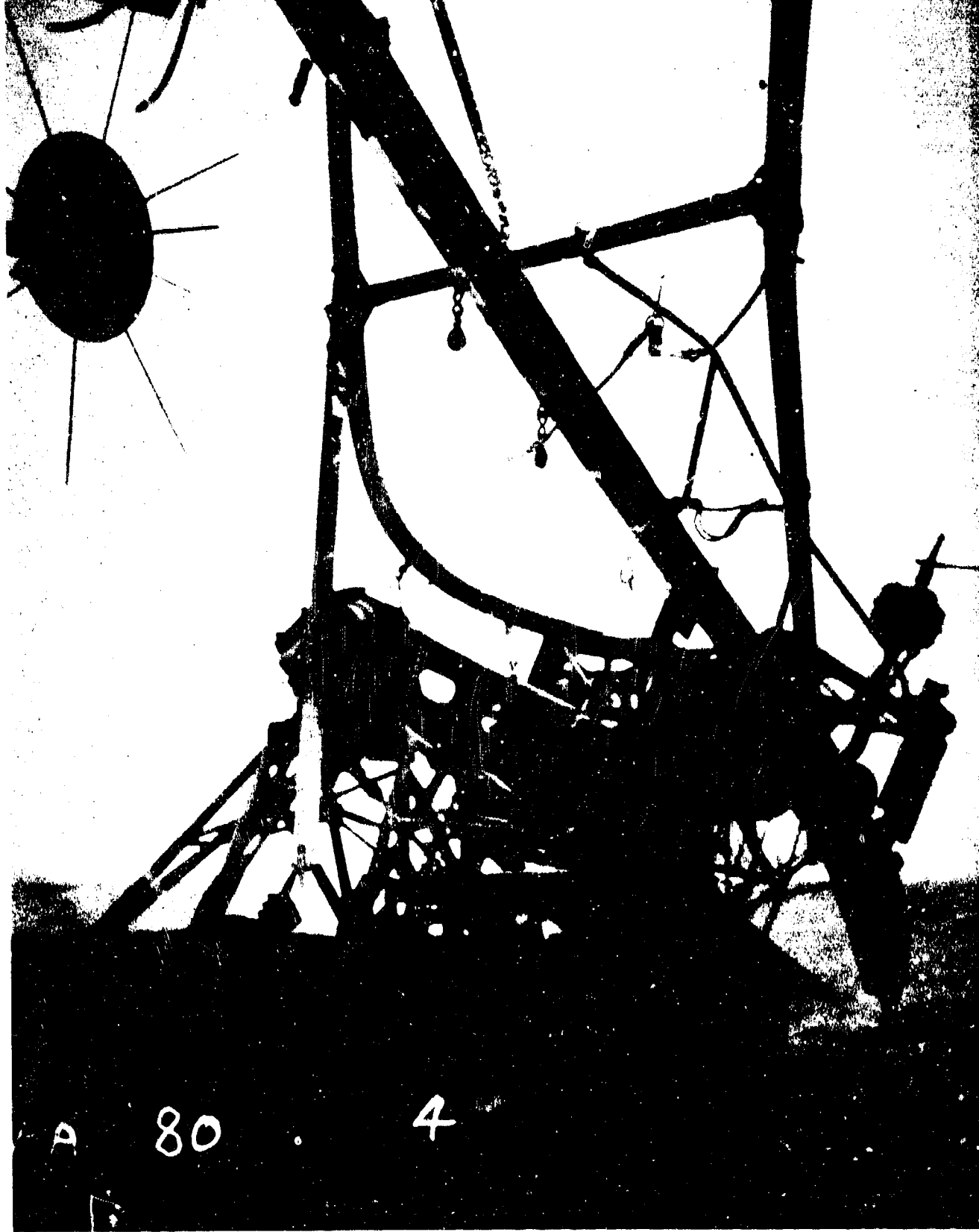
AA-CR-80-1900-4. USS NEVADA (BB36). Forward tripod, view looking forward at wreckage of starboard yardarm. Main member, truss and forward strut.
