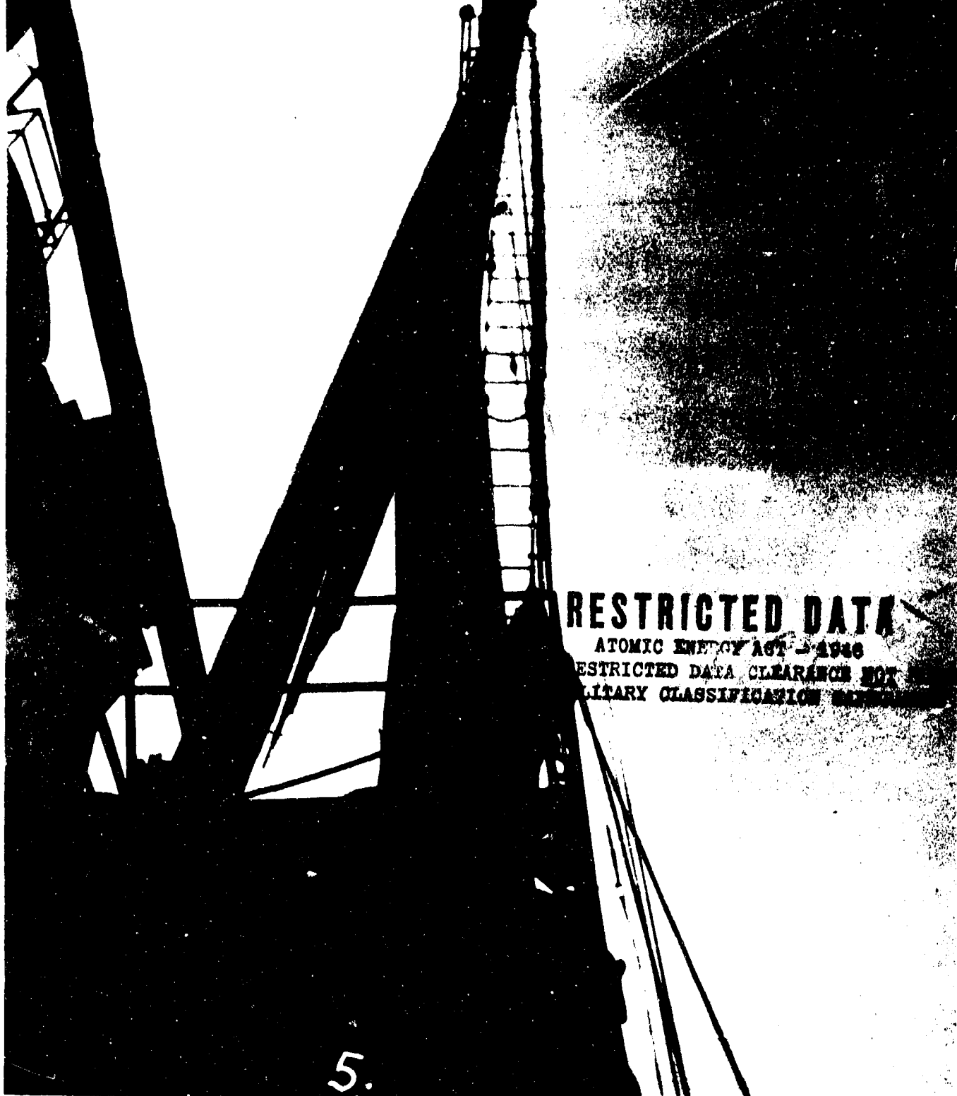
AA-CR-92-1774-5. PRINZ EUGEN (IX300). Broken mast, looking up, after Test Able.
